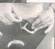
Mount tweeter and mid range speakers. Connect the faders, seat them and screw into position. Note the use of a gasket (above) for prevention of air leaks.
